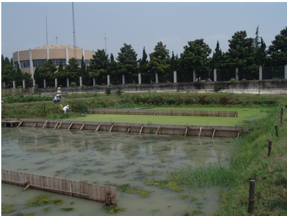
Figure 7: Green Liver System® constructed at the water work facilities of Hefei City at Lake ChaoHu (PR China) consisting of six compartments: 1+2 covered with Lema minor ; 3+4
